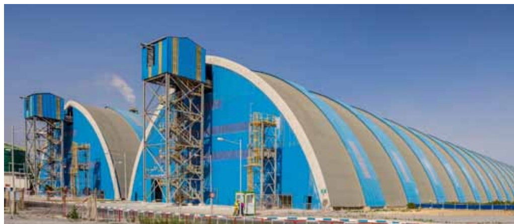
Halls de stockage ODI- OCP Jorf Lasfar
